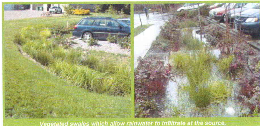
Vegetated swales which allow rainwater to infiltrate at the source.
