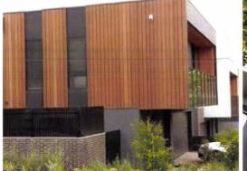
Innowood Composite timber cladding to spandrel panels
