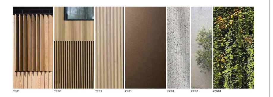
TC01 - TIMBER CLADDING 600mm CENTRES 250mm PANEL TC02 - ALUMINIUM PROFILE PANEL TC03 - FIBRE CEMENT PANEL WITH APPLIED FINISH CL01 - ALUMINUM CLADDING (COLOUR INDICATIVE) CC01 - TEXTURED CONCRETE PANEL CC02 - TEXTURED CONCRETE RENDER GW01 - PANELISED GREEN WALL SYSTEM
