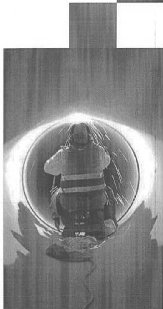
A welder inside one of the pipelines at Thomsons Reservoir. Water from the Perth Seawater Desalination Plant is stored at the reservoir before being transferred, via the Nicholson Road pump station into the IWSS.
