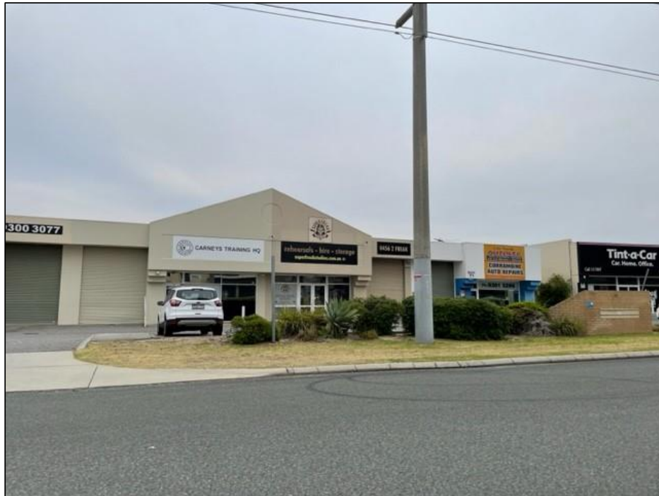
Figure 6- 71 Winton Road, Joondalup
