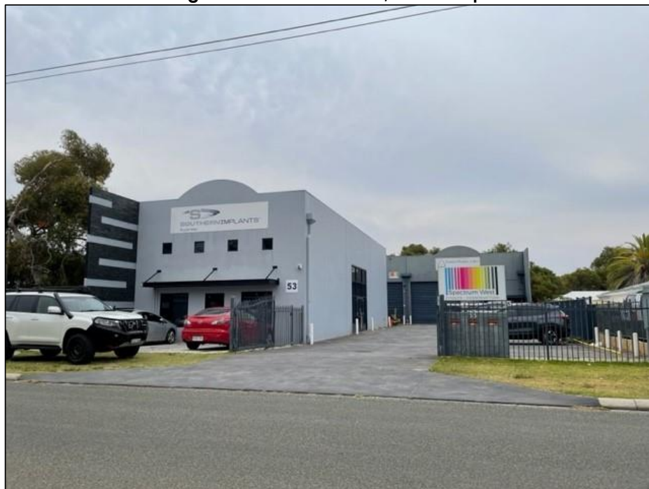
Figure 7 – 53 Winton Road, Joondalup
