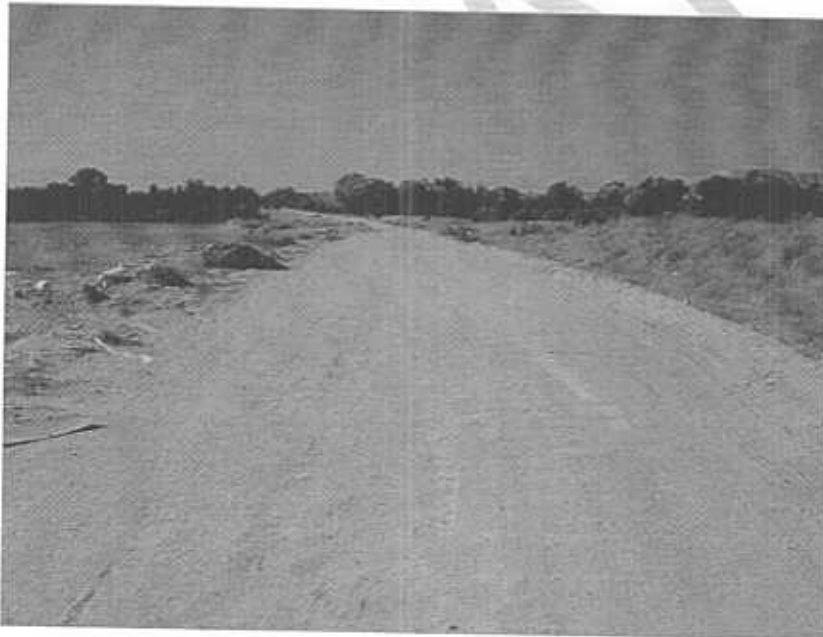
Figure 9: Connolly Drive extension -limestone stage
