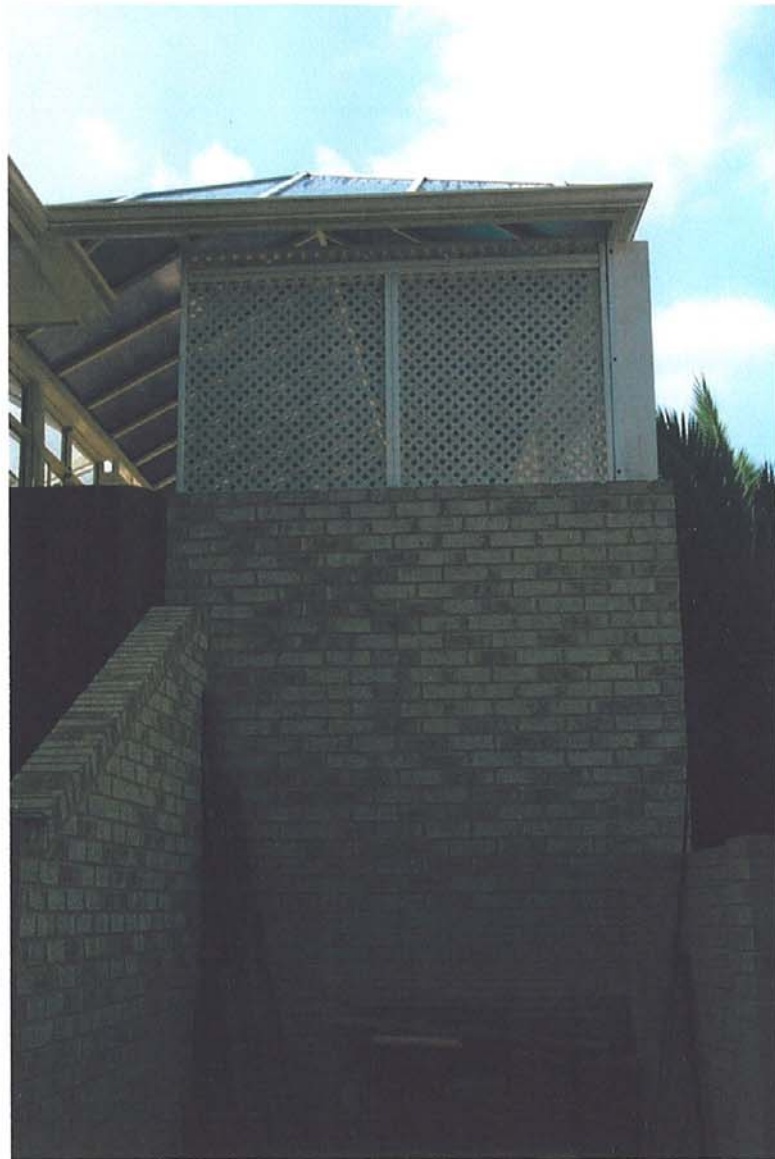
Figure 1: Patio (not pergola) has been constructed to Southern side of property. Adjoining property is set significantly lower.
