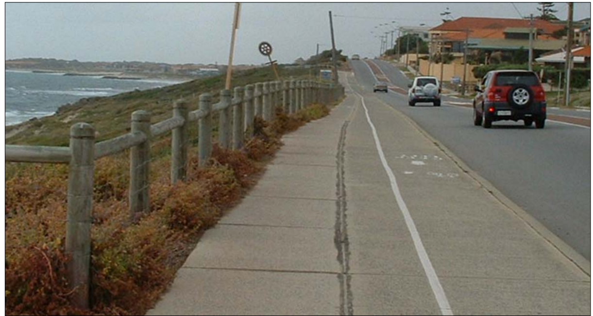
Existing condition of the dual use path.
