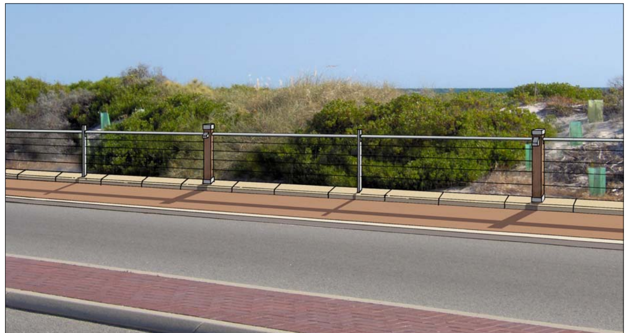
Proposed fencing design and improved dual use path showing relationship to dunes and adjacent vegetation.
