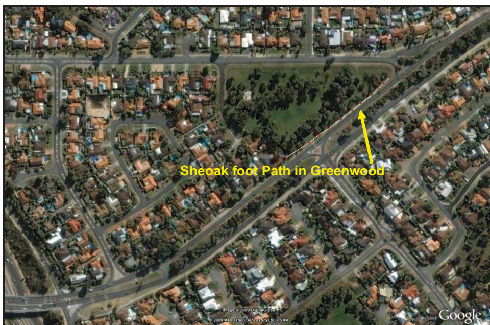
Figure 4 shows the Sheoak site in Greenwood. At this location there is a footpath on Warwick road and a 3 cm strip to either side of the footpath including joins was treated.
