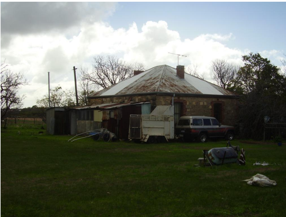
Rear (west) of Jack Duffy House , showing lean-to extension and outside toilet (July 2009)
