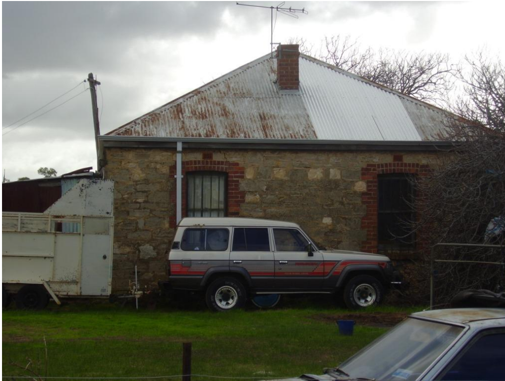
South façade of Jack Duffy House , showing quoining at windows (July 2009)
