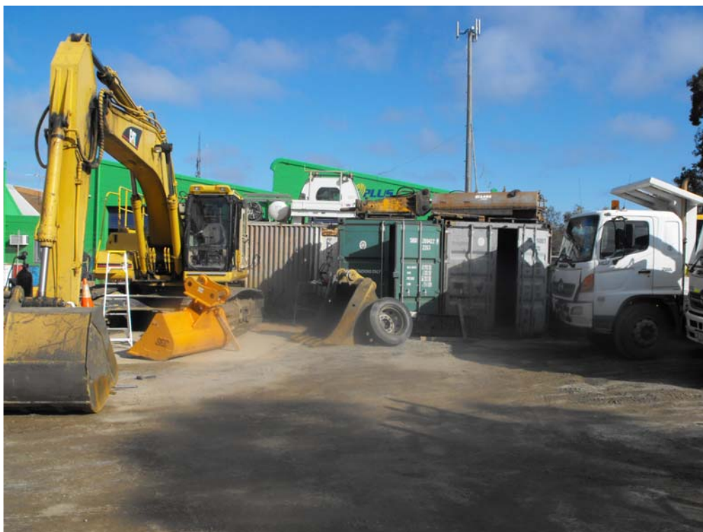
Photo 4 – Equipment and materials stored on site
