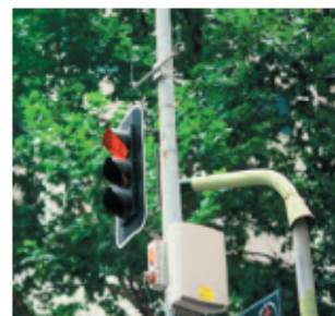
Microcell Mounted on Traffic Lights
