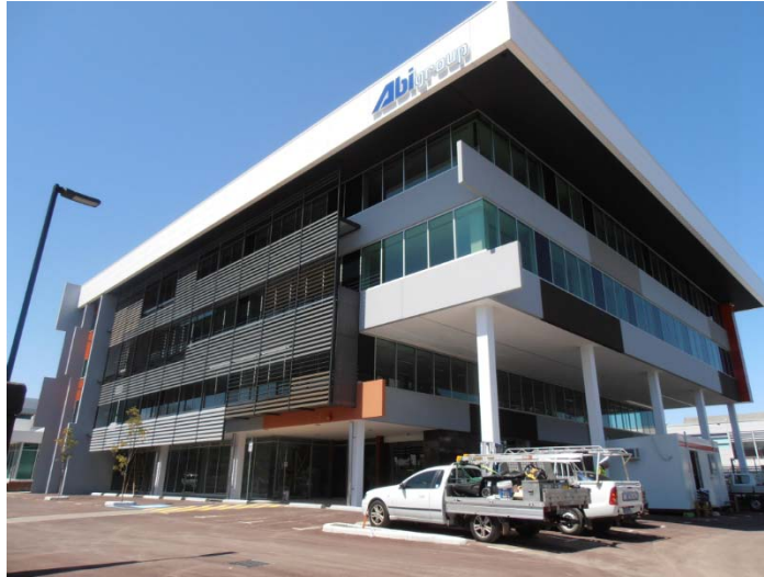
Figure 18 East Link Office Park (WA)
