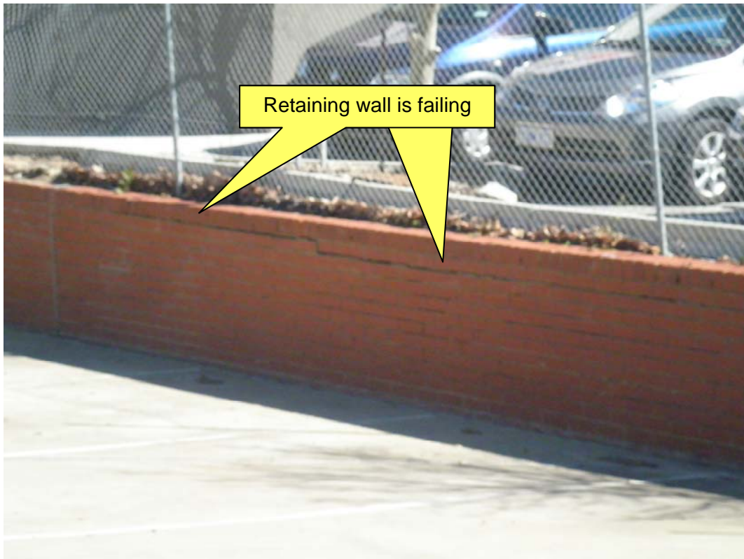
Photo shows the existing retaining wall is failing.
