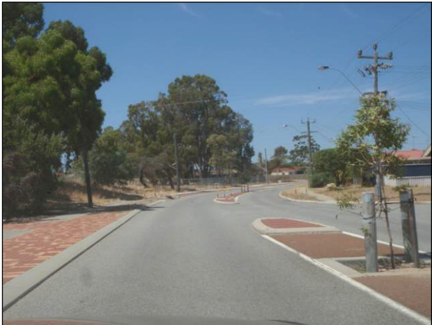
Camberwarra Dr, looking east towards Fenellia Cres
