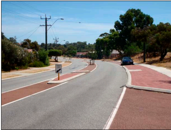
Photo 11: Approximate sight lines from Road 2 along Camberwarra Dr to the west
