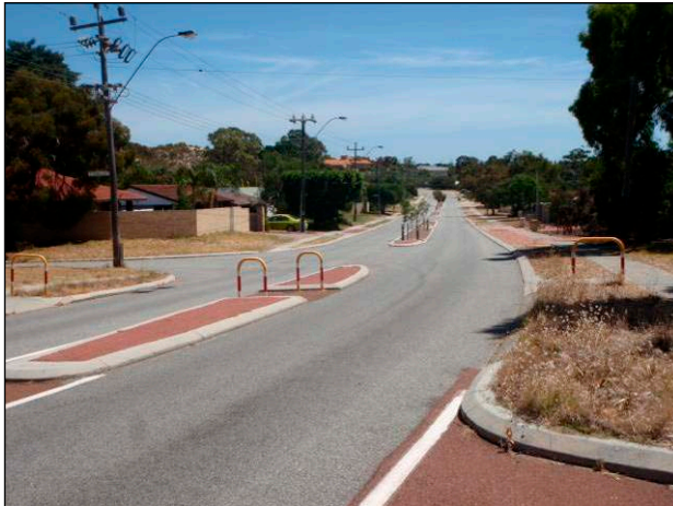
Photo 9: Approximate sight lines from Road 1 along Camberwarra Dr to the west
