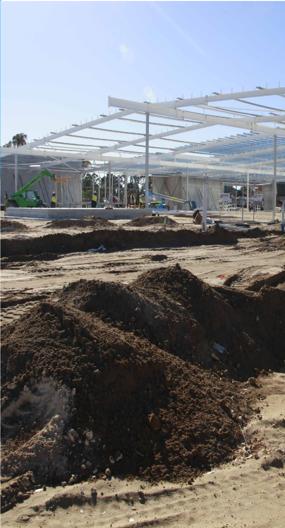
Joondalup Quadrangle construction
