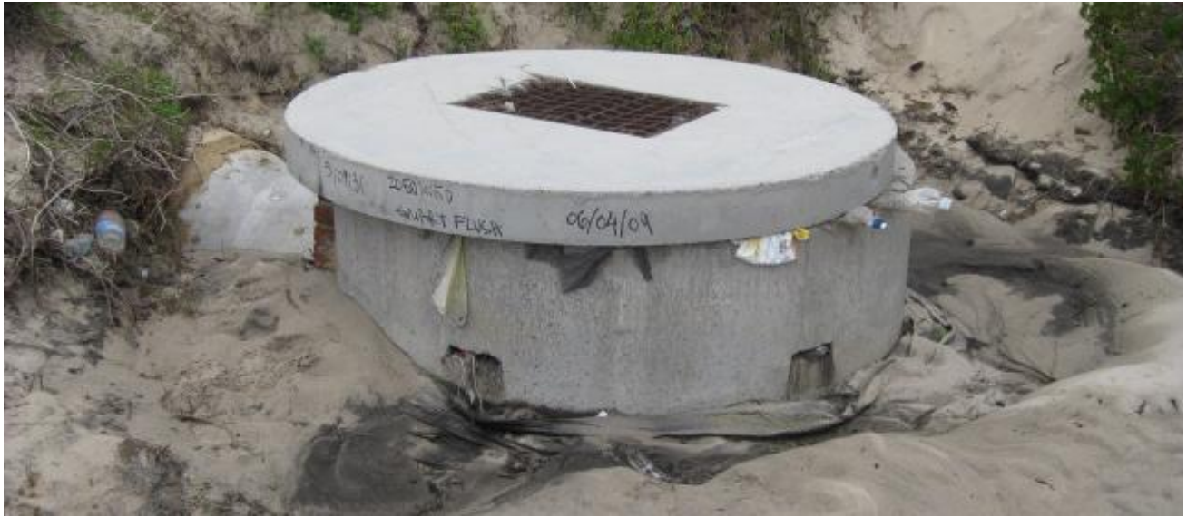
Figure 25: Drain lid movement caused by storm surge and expelled rubbish (Photo © M. Norman)
