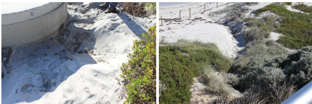
Figure 6: Erosion around stormwater drains creating gullies towards the beach within the site
