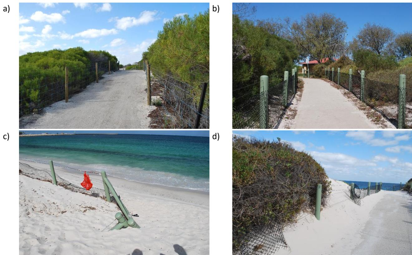
**Figure 20:** Fencing: a) pine post and square ringlock and wire fencing, b) PVC sleeves over pine posts and chainmesh fencing, c) fencing buried due to coastal erosion of sand dunes, d) fencing damaged along beach access path.
