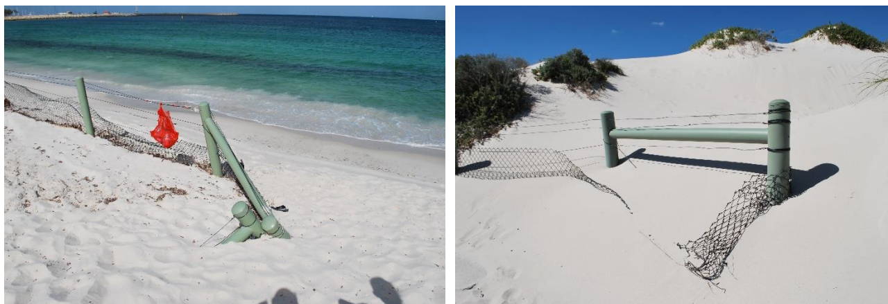
Figure 6: Erosion along the foredunes and beach affecting stability of fencing
