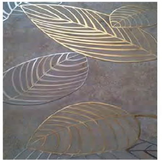
Example of steel inlay in concrete
