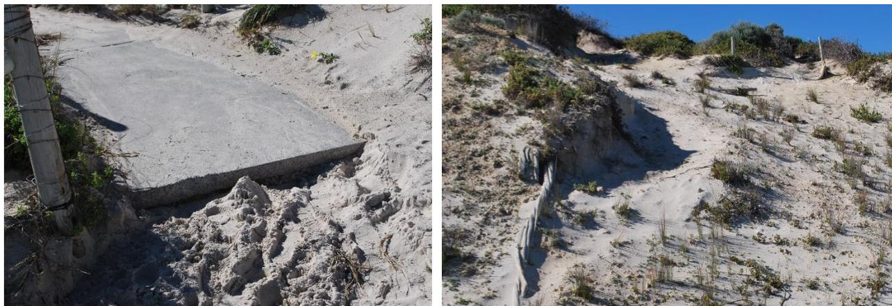
**Figure 6:** Erosion at the end of a concrete path and on higher foredunes in the south-west of the Reserve
