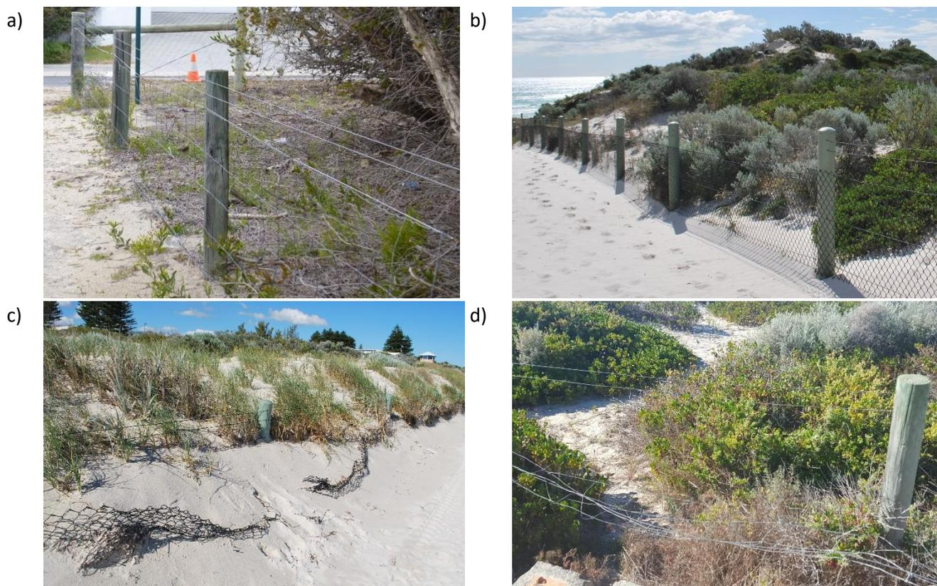
**Figure 20:** Fencing: a) pine post and square ringlock and wire fencing, b) PVC sleeves over pine posts and chainmesh fencing, c) damaged fencing along the beach d) damaged fencing adjacent access way.
