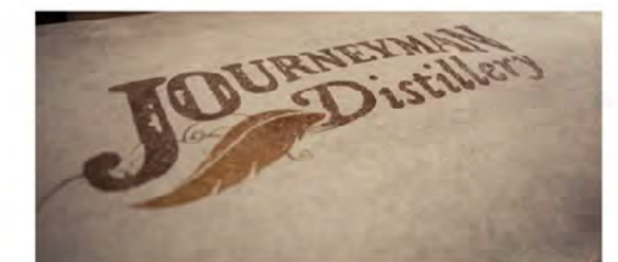
Example of wording etched into concrete
