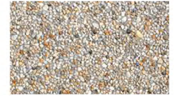
Example of exposed aggregate concrete
