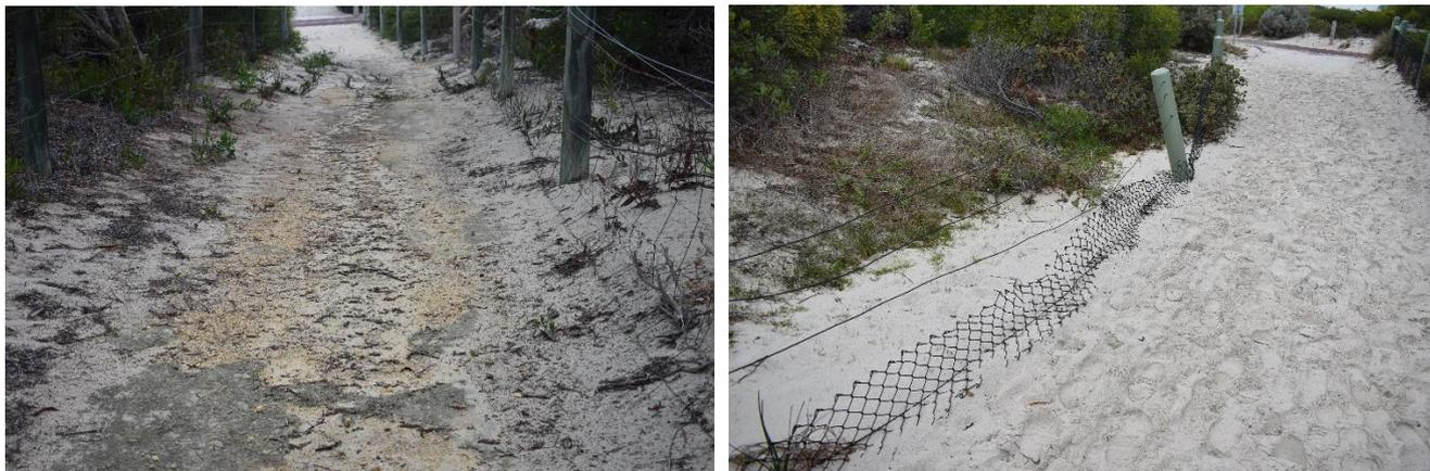
**Figure 23:** Pathway requiring maintenance (left), and subject to erosion (right)
