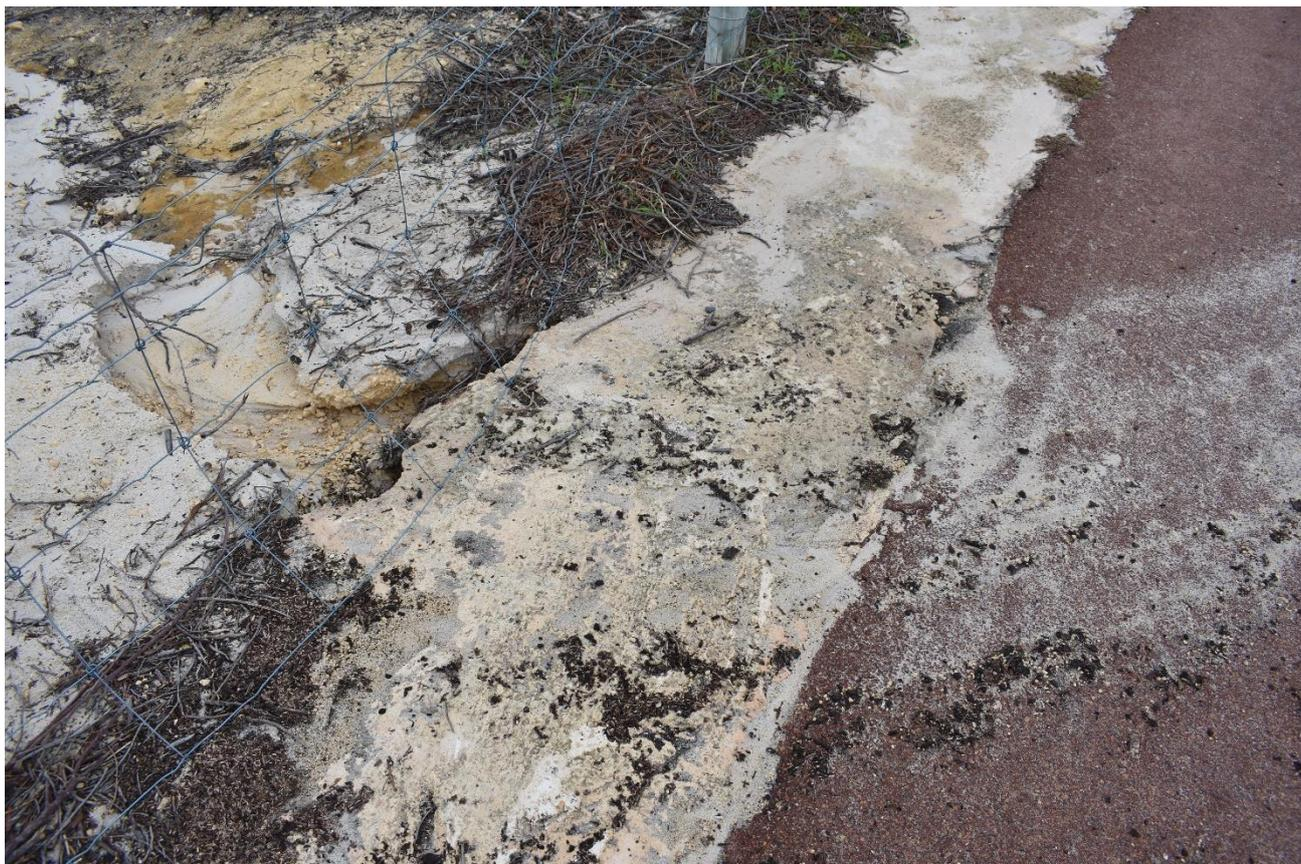
**Figure 6:** Runoff causing erosion off the dual use path into the adjacent dune swale
