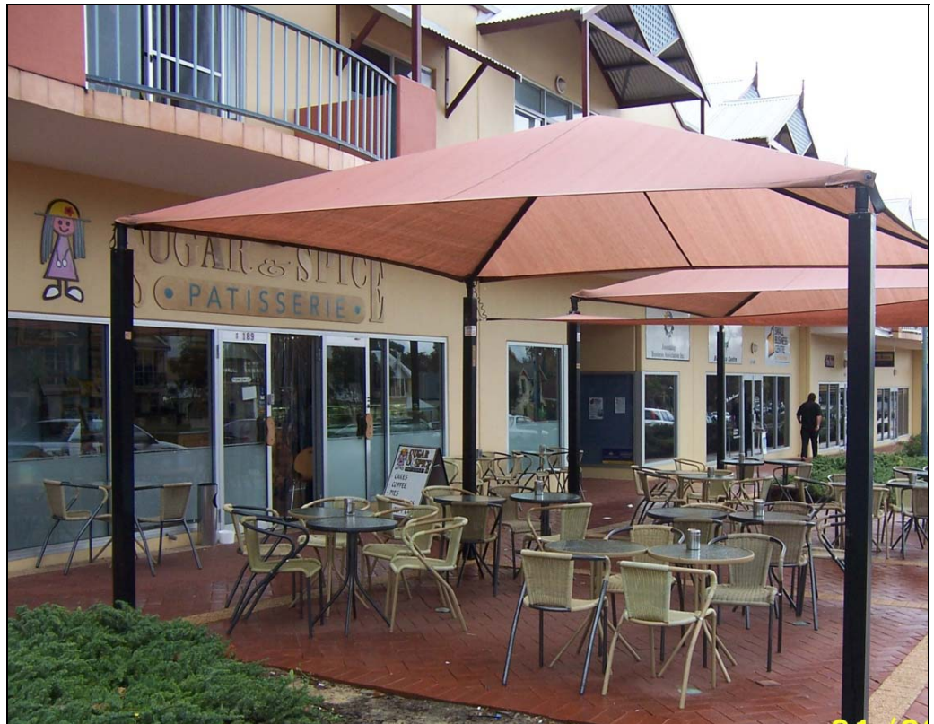
Figure 5. Example of a permanent shade structure on 9 metres wide verge.
