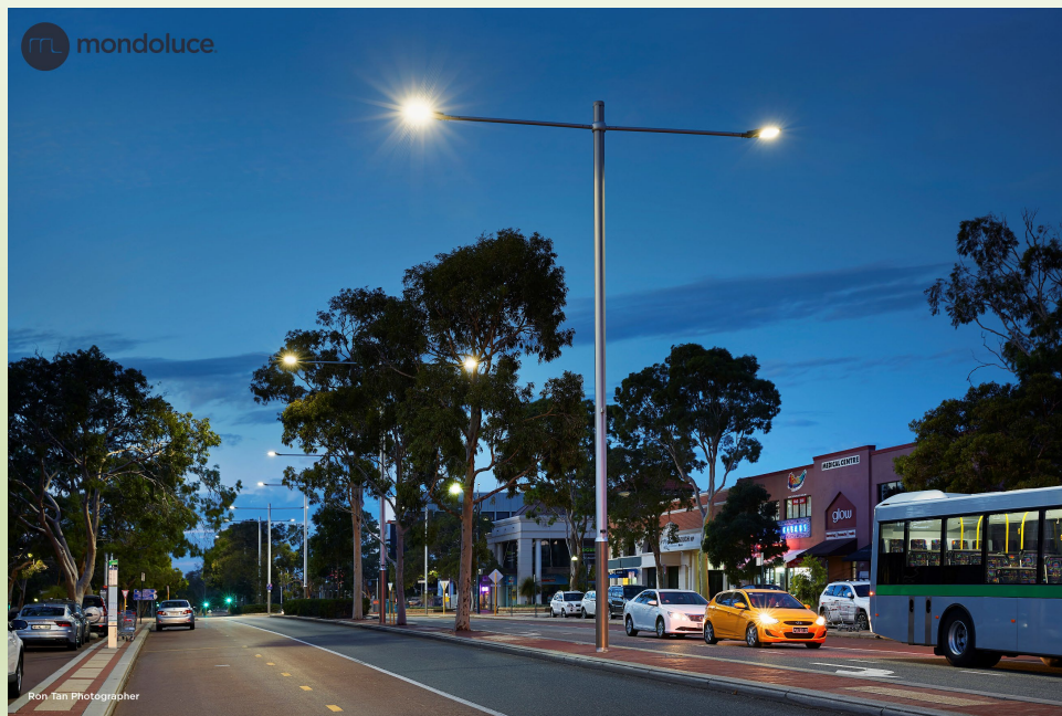
Energy efficient LED lighting in Joondalup
