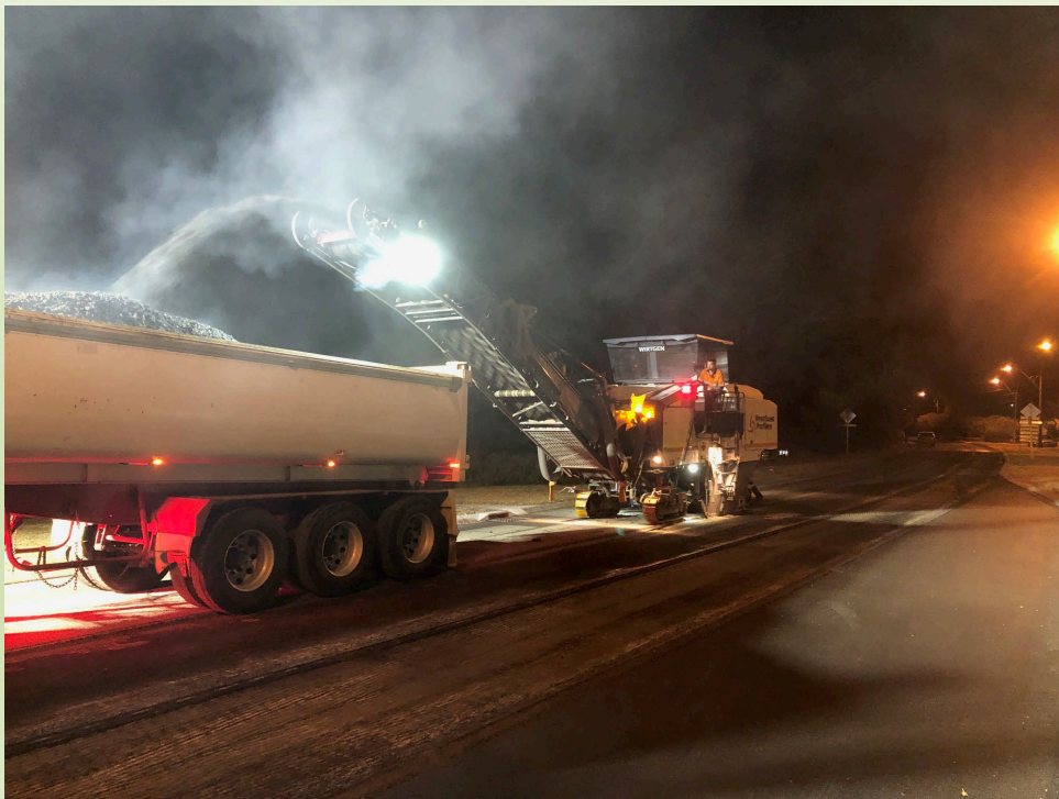
Road upgrade using recycled waste
