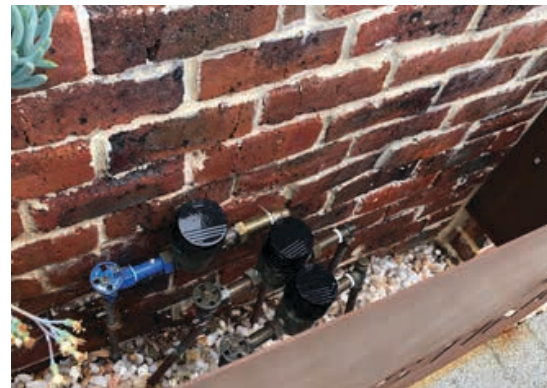
Photo G2.5a and b Effective screening of water meters within the front setback area of this development reduces visual impact and allows for easy access and maintenance when required
