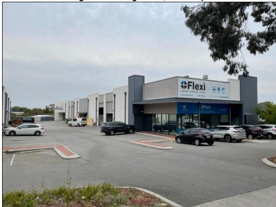
Figure 5 – 21 Delage Street, Joondalup
