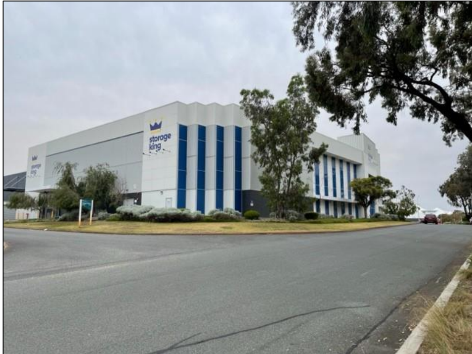
Figure 4 – 2 Delage Street, Joondalup
